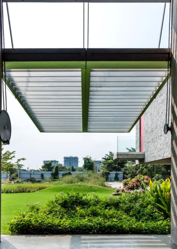
THE LOUVERED FAÇADE
