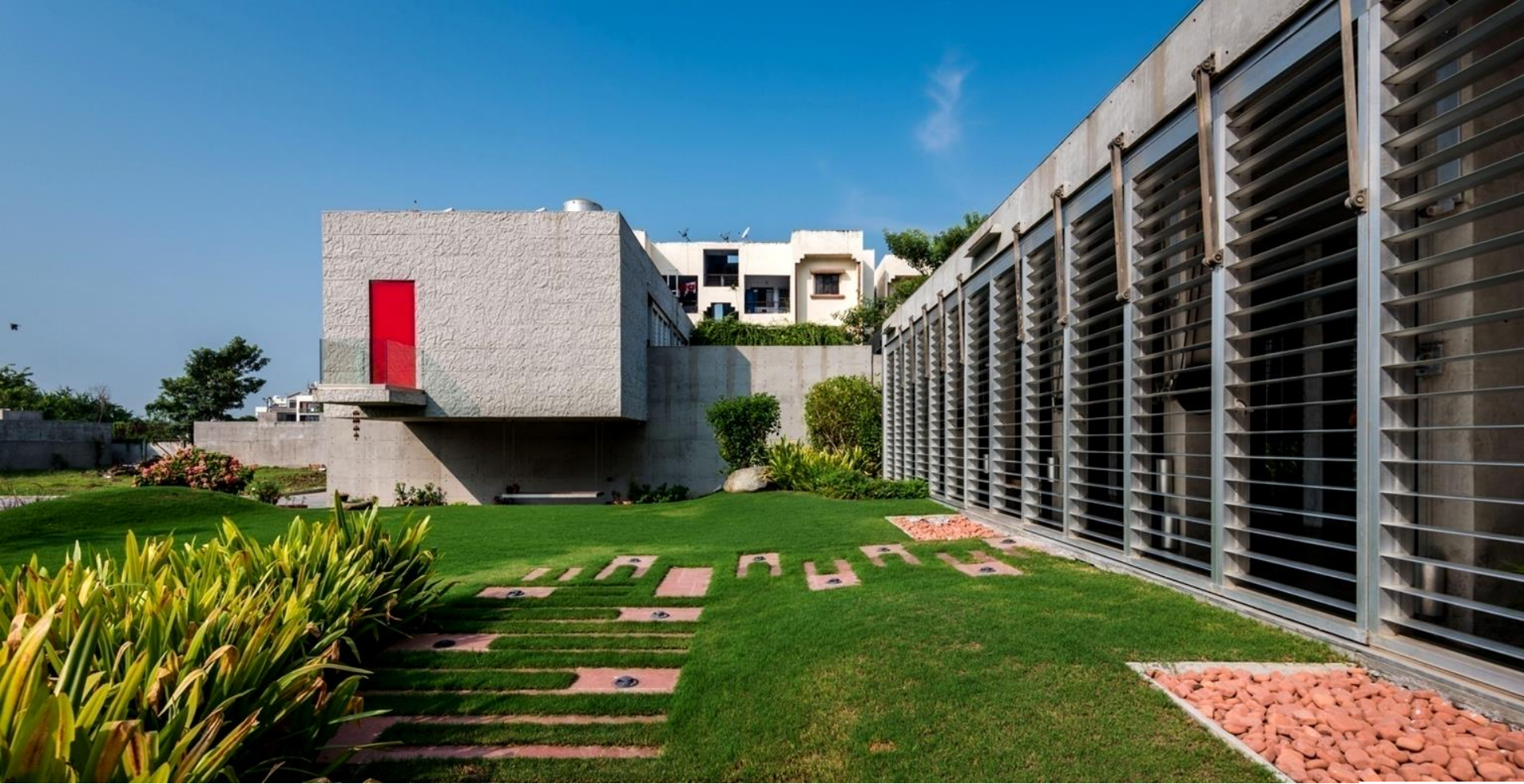
THE FAÇADE WITH THE UNIQUE LOUVERS MECHANISM
