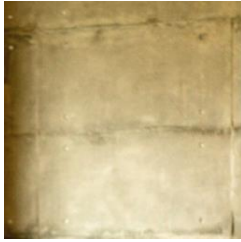
FORM FINISHED CONCRETE
