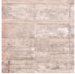
FORM FINISHED CONCRETE
